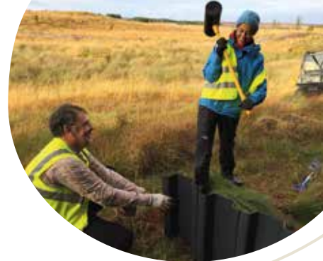
Creating dams, to restore the water table Image: Paul Turner, RSPB
